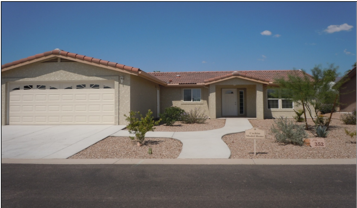
Example of tile roofing and stucco siding added after delivery of manufactured housing
